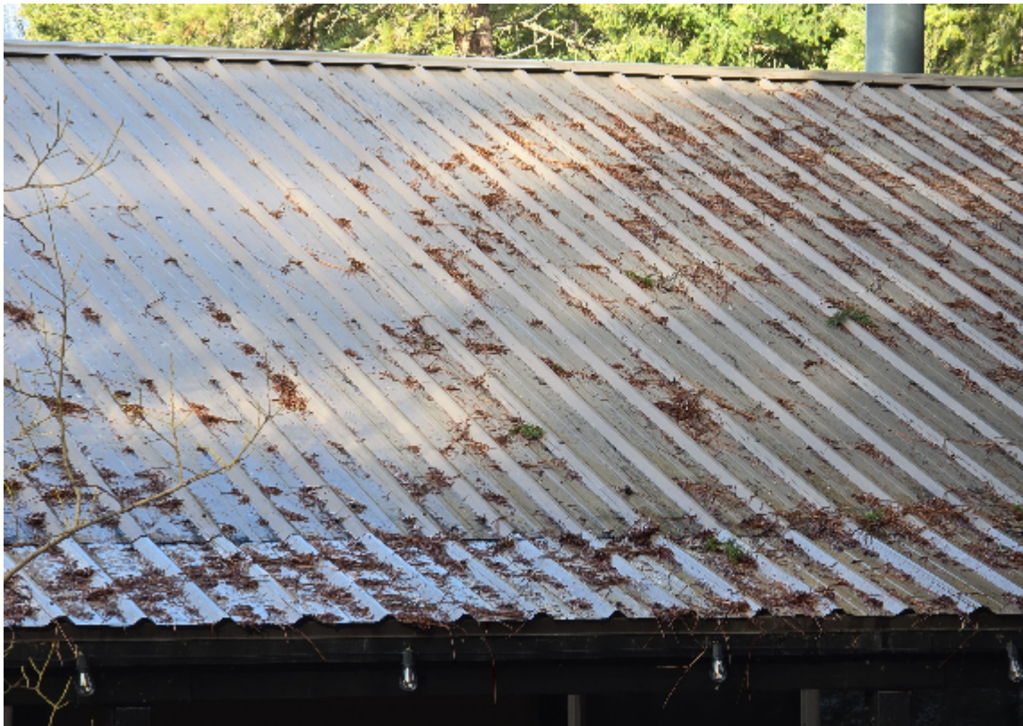
Building Exterior - Roof, Metal Standing Seam
