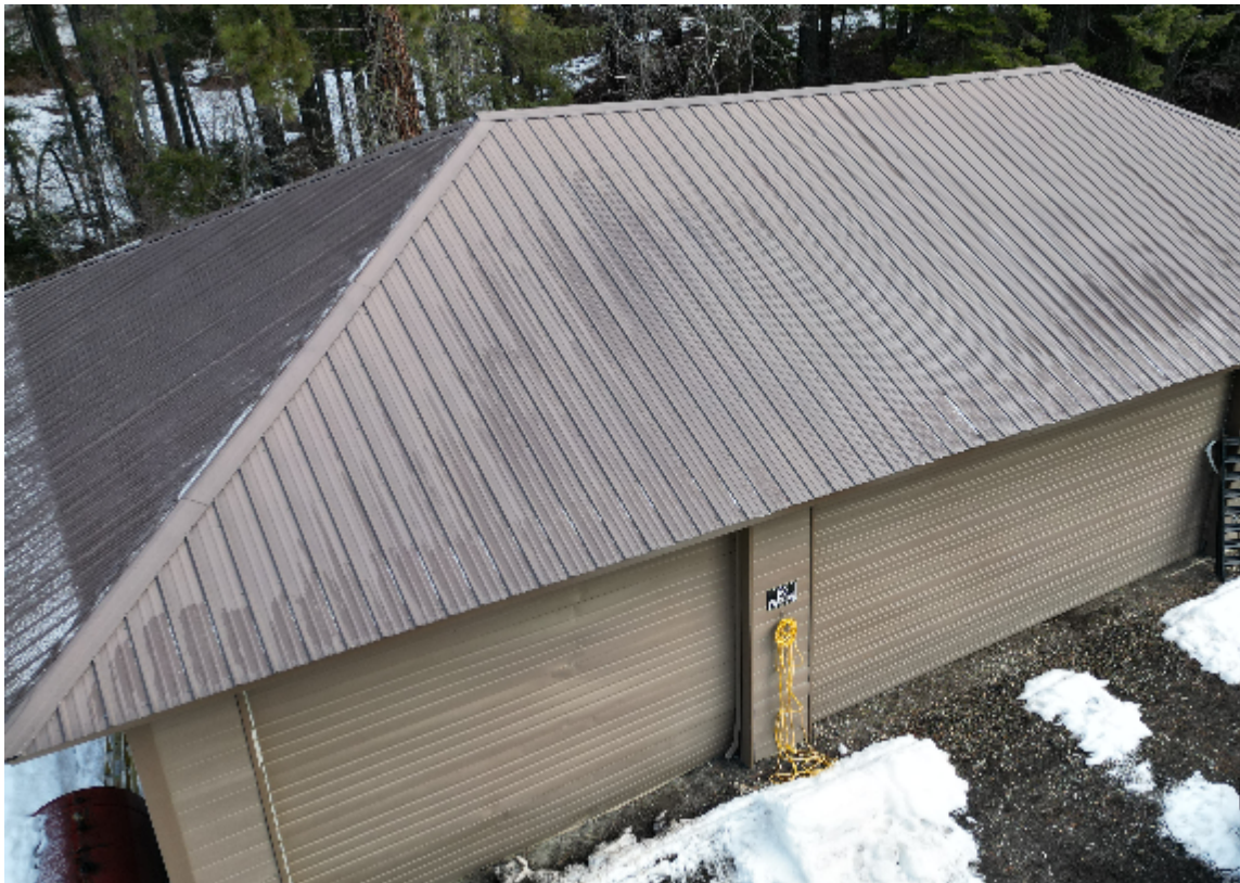
Building Exterior - Roof, Metal Standing Seam
