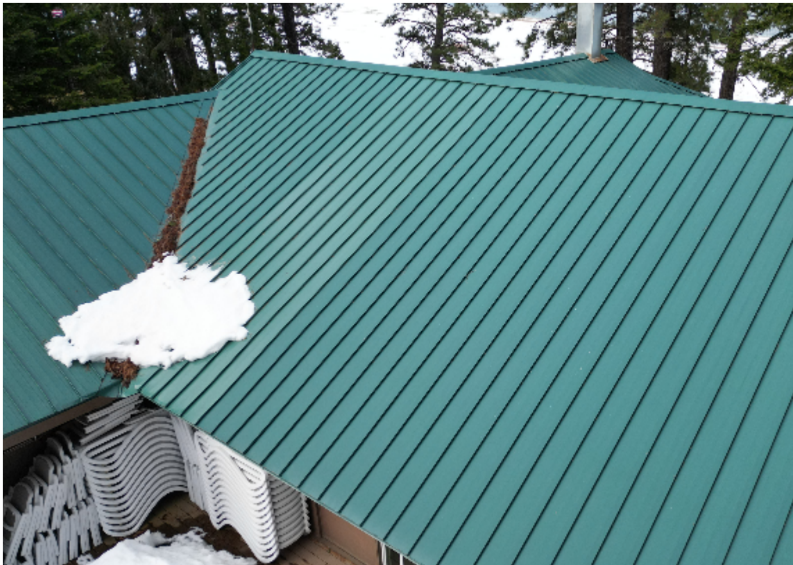
Building Exterior - Roof, Metal Standing Seam
