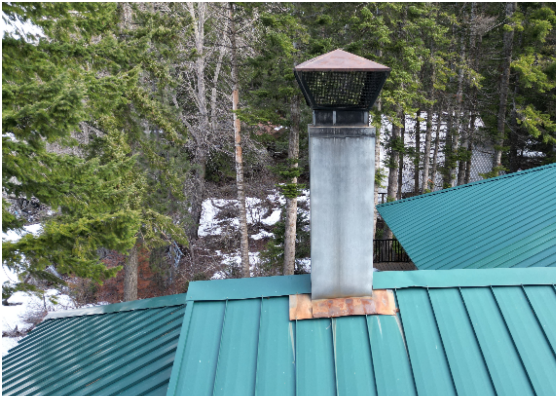
Building Exterior - Flue/Flue Caps
